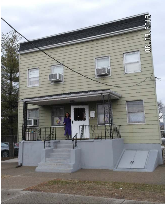
Front elevation of 32 Sherwood taken from access road to parking garage
