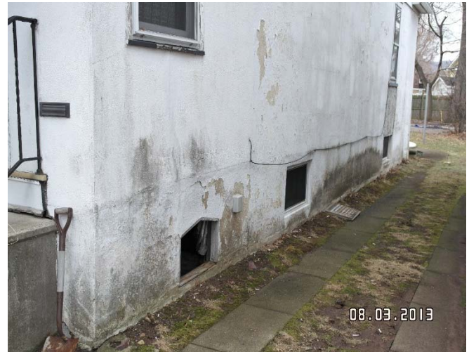
View of right elevation, exterior mold, evidence of repairs to foundation and missing basement window.
