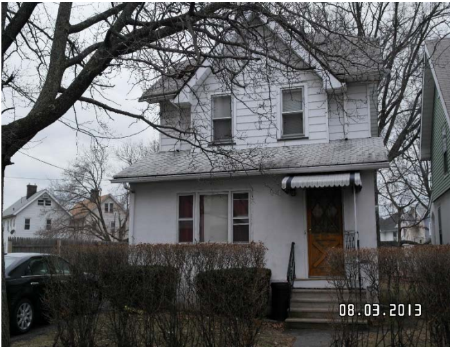
Front elevation of 16 Walnut Crescent
