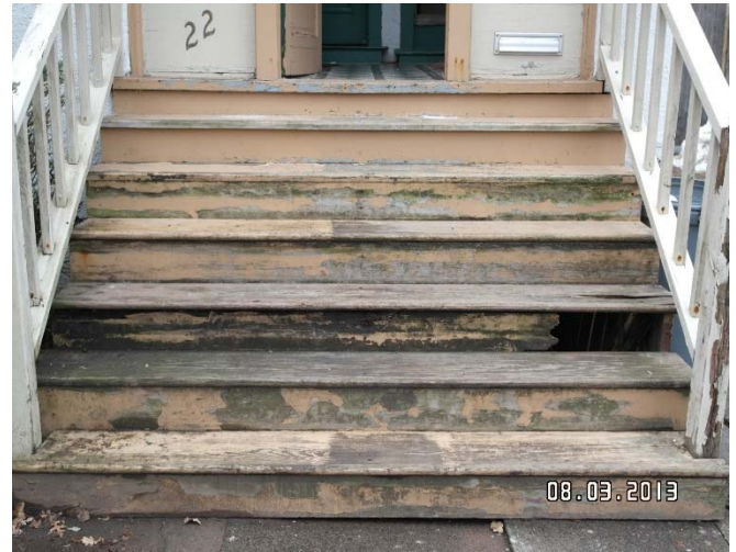
Front steps in poor condition, rotted wood and missing riser
