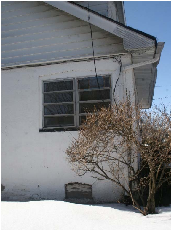
Boarded up basement window on left elevation of house
