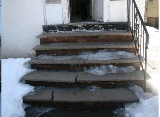
Evidence of broken front steps
