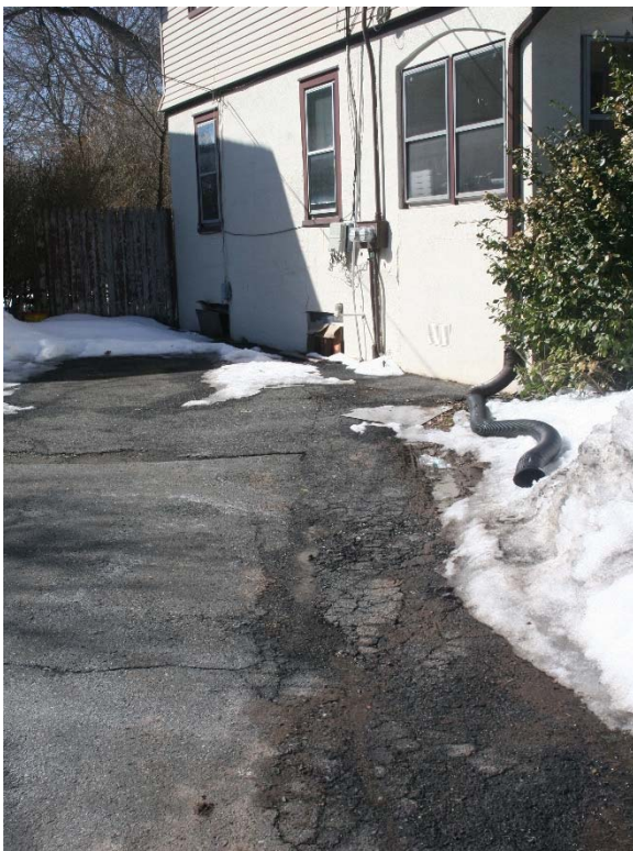
Boarded up basement windows along front right elevation. Driveway in poor condition
