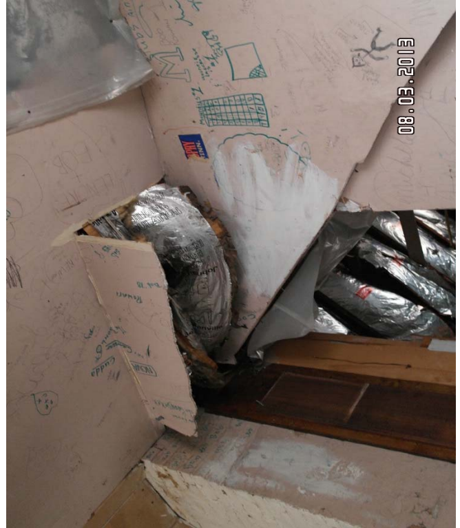
Close up image of plastic sheeting on hallway ceiling and exposed insulation
