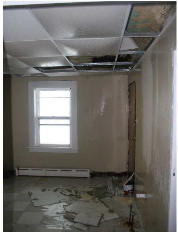
View of kitchen from living room. Drop ceiling collapsed from water damage. Water leaking through 2 nd floor
