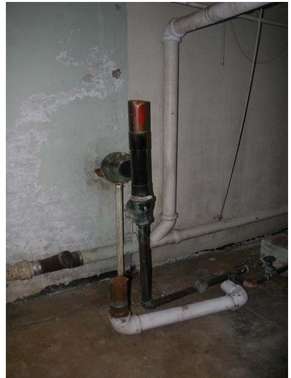
Disconnected Sewer lateral
