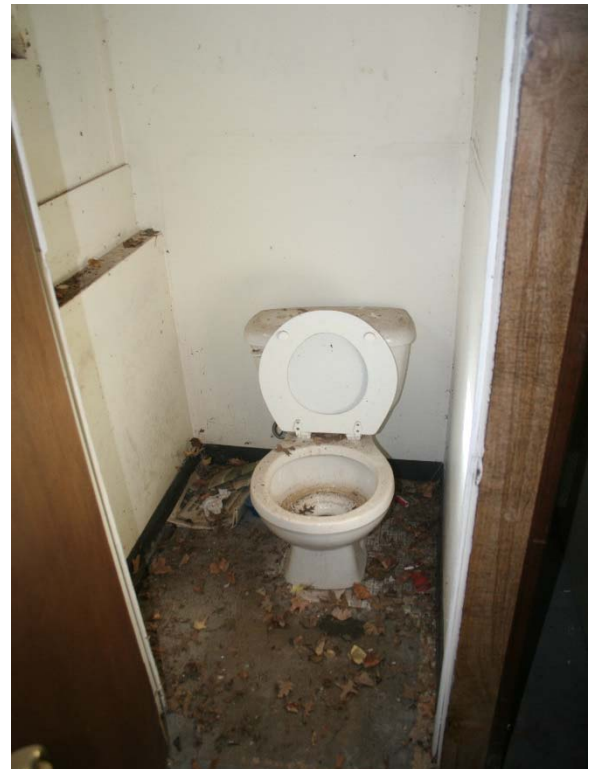
Evidence of water damage on floor and broken toilet
