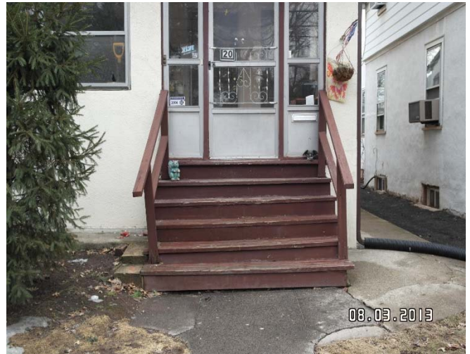
Entrance to house in poor condition
