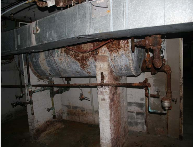
Utilities/ductwork in basement area.
