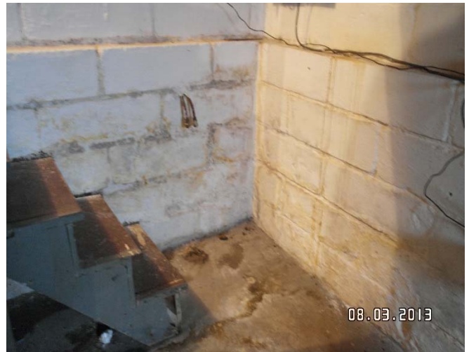
Steep steps heading down to basement, with no support railing
