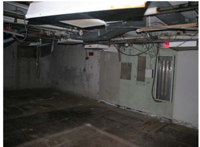
Old office space after removal of asbestos tile and drop ceiling
