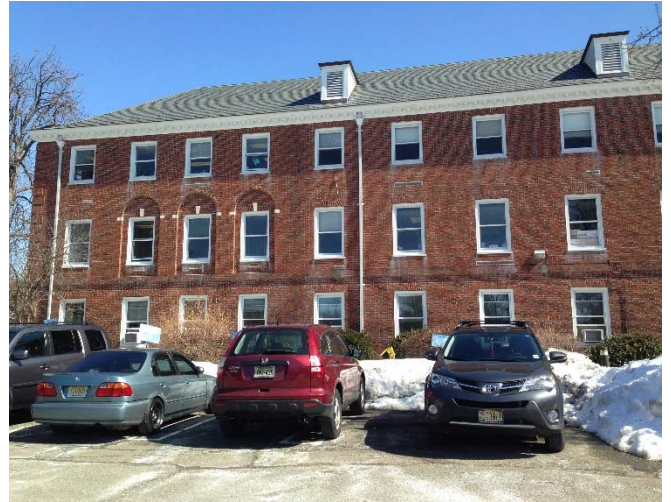
Handicap spaces that do not meet regulations as they are missing access aisles
