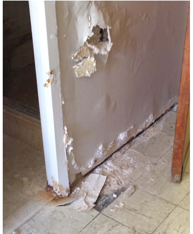
Water damaged wall, adjacent to shower in dormitory room (typical)
