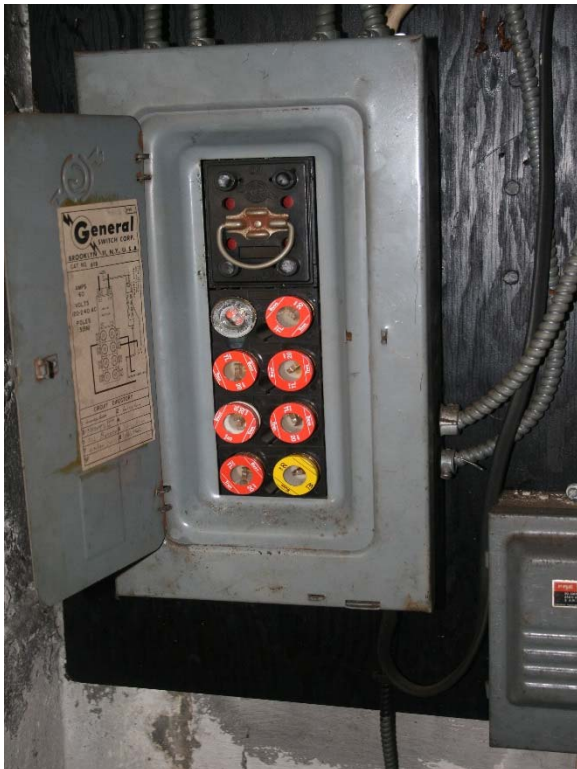
Knob and tube electrical box, does not meet current code standards
