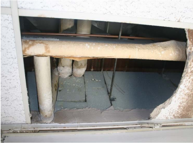
Ceiling opened up for asbestos testing
