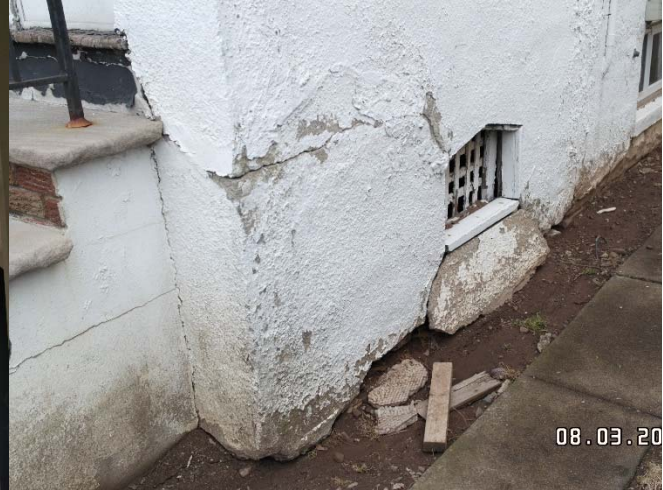
Structural damage along front right elevation adjacent to front steps
