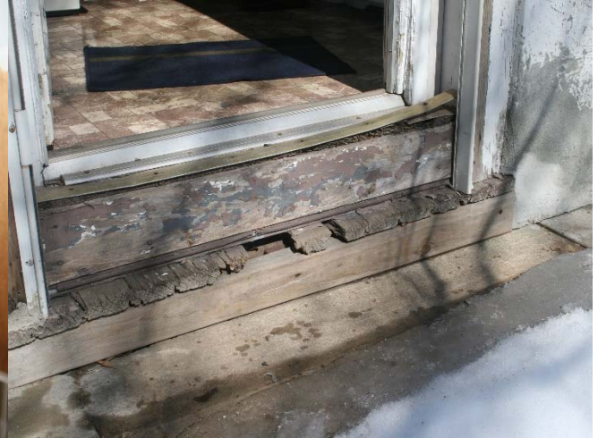
Evidence of rotten sub floor on rear entrance to structure as entering the kitchen
