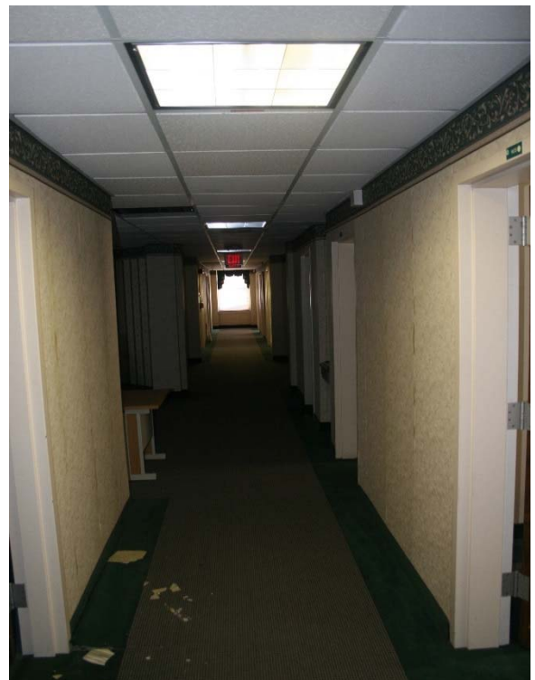
Hallway leading to additional offices
