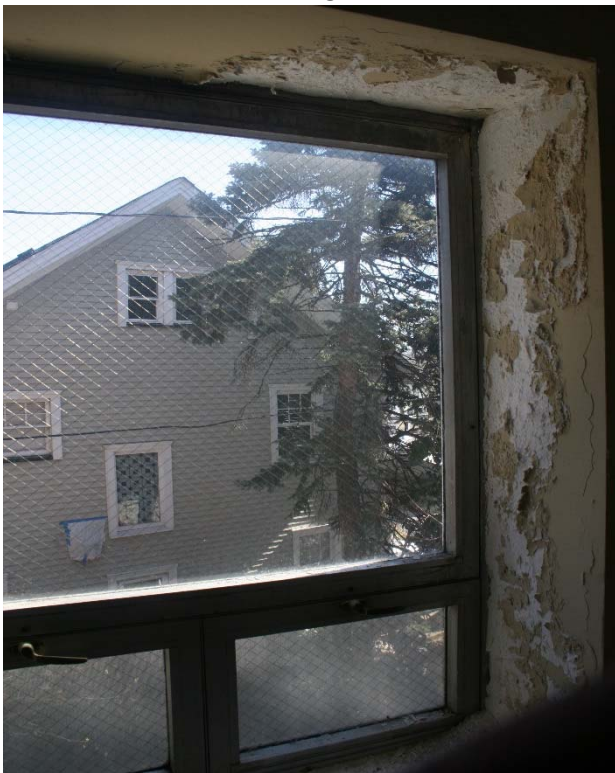
Water damage around windows
