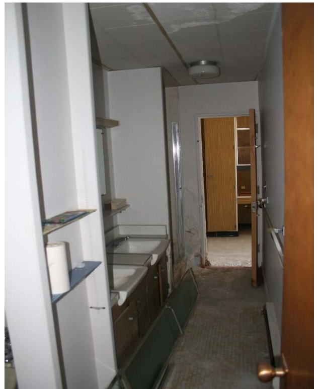
View of bathroom that is shared by two adjacent rooms or four nursing students
