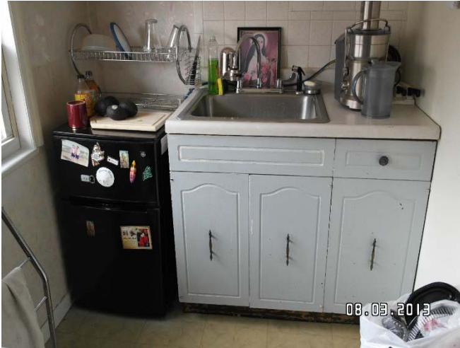
Small ½ kitchen on illegal 3 rd floor unit
