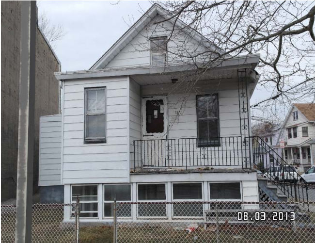
Front elevation of 34 Sherwood
