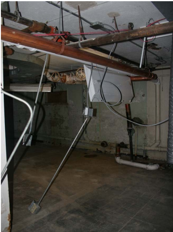
Looking at old lighting for office space
