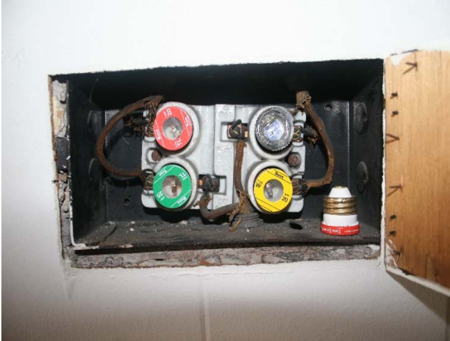
Knob and tube wiring in main entranceway of structure. Does not meet current code standards
