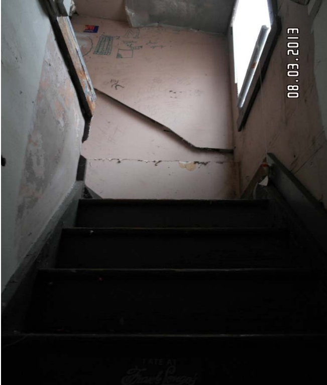
Hallway at top of staircase, walls in poor condition. Plastic sheeting on top ceiling where water damage occurred.
