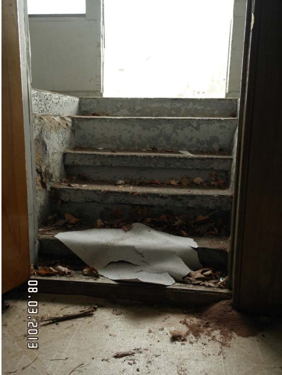
Entrance to basement
