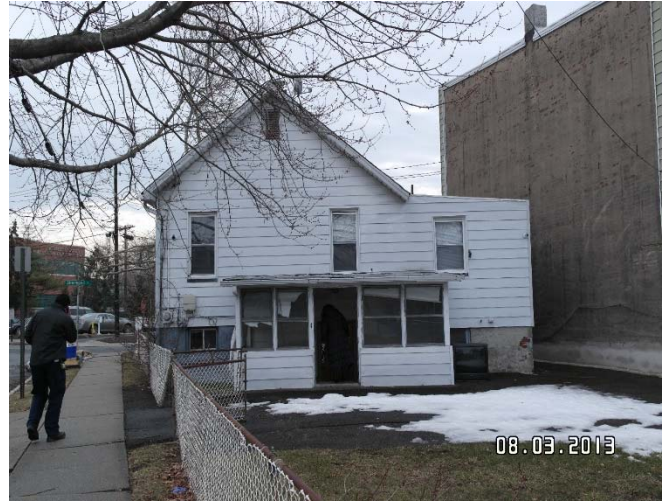
Rear elevation of property
