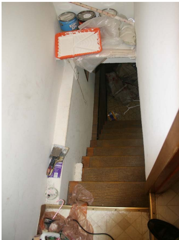
Very narrow & steep staircase to basement, no handrail. Difficult access.
