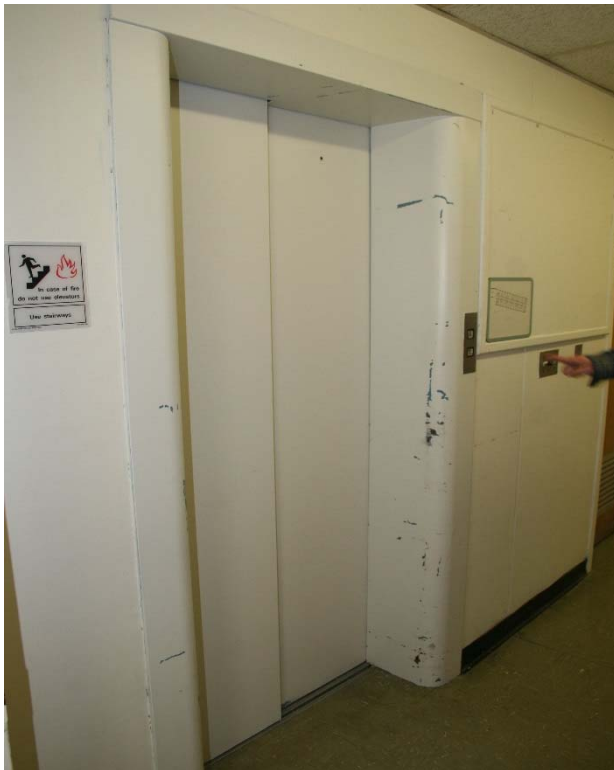
Single small elevator at main entrance to building
