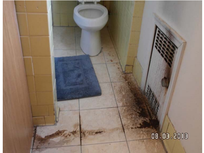
Upstairs bathroom with rusted radiator cover, evidence of water leak.
