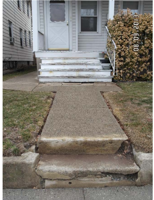
Broken concrete of front entrance walkway
