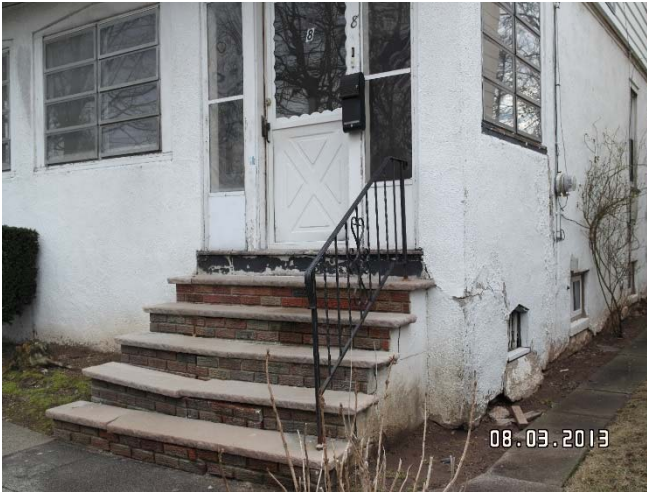
Additional view of damage to front steps and front right corner of house
