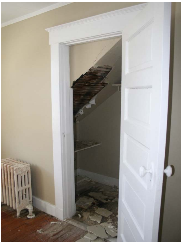
Water damage along 2 nd floor ceiling in bedroom closet
