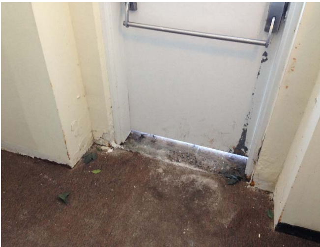
Exit door. Water floods under doorway
