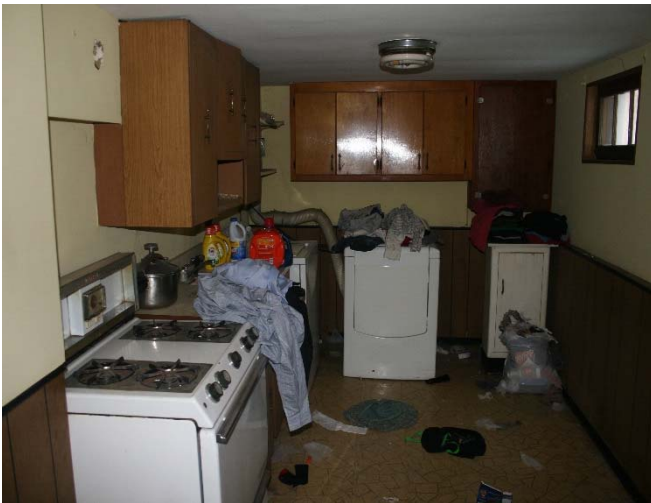
Illegal kitchen set up in basement. Does not meet building code standards.
