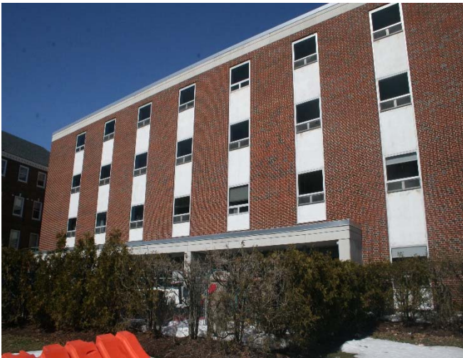
Looking at front façade of Nursing School Dormitory
