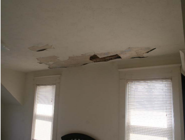
Water damage along ceiling on 2 nd floor bedroom
