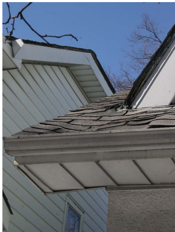
Evidence of rotting roof and shingles on the front left edge of the roof
