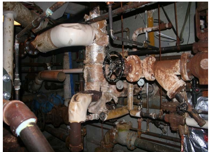
Valves for hot water supply pipes
