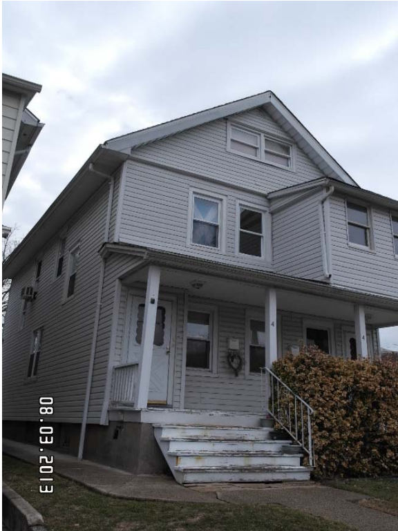
Front elevation view of 4 George Street
