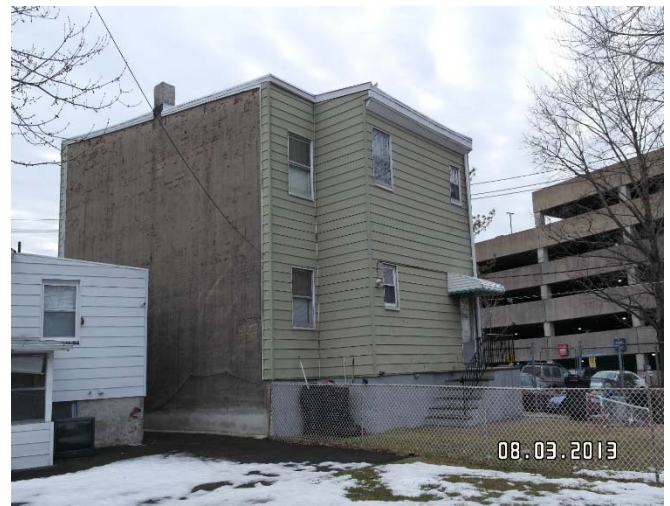
Rear view of property shows no parking garage and windowless right facade
