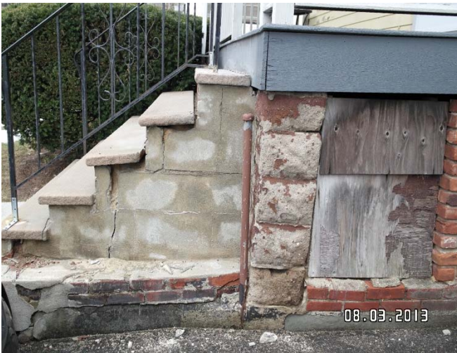
Evidence of cracking on front steps with masonry and brick work repairs
