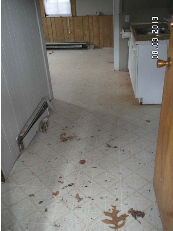
View of kitchen and non-operational baseboard heating
