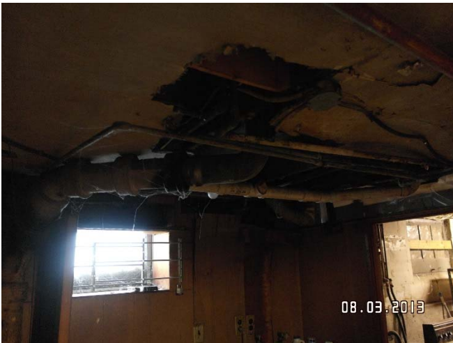
Basement ceiling falling apart along water pipes leading upstairs
