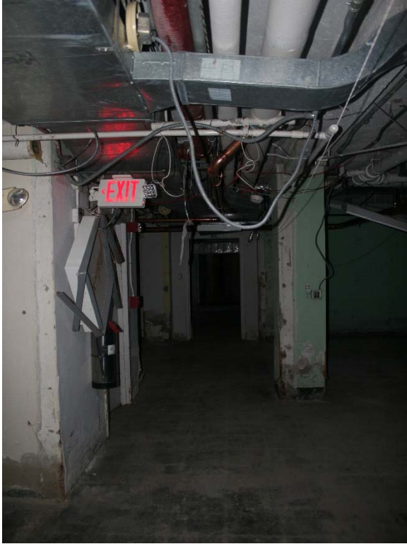
Utilities at the entrance to the old offices located in the basement
