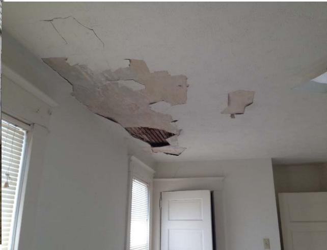
Evidence of leaking roof in front bedroom
