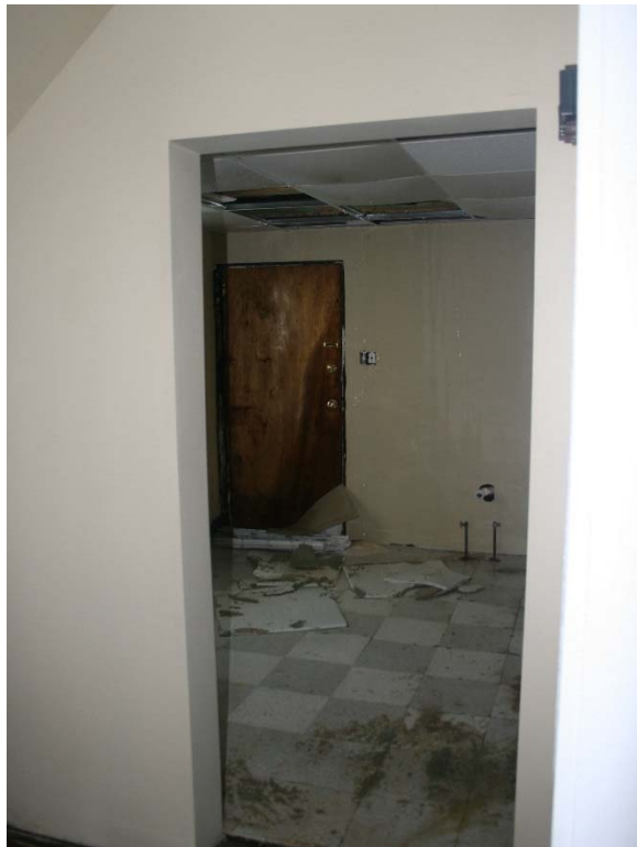
View of kitchen are from front entryway. Kitchen does not contain any appliance or cabinets and is non functional
