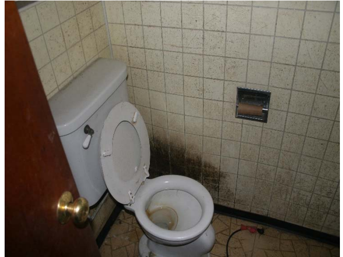
Interior bathroom with lack of maintenance and mold on wall and floor.
