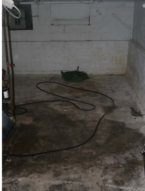
Evidence of water damage in basement
