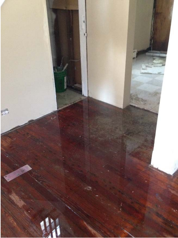
Ponding water in front foyer from leaky 2 nd floor pipe. Looking at basement entrance with no door
