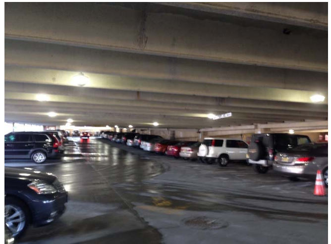
Interior view of parking structure parking bay
