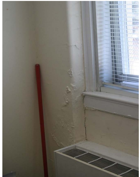
Evidence of water damage along window frame edges. Typical of most offices.
