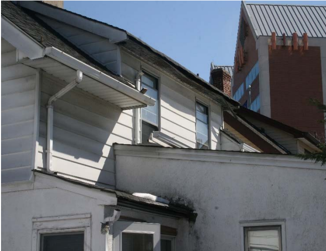
Close up of missing roof tiles and missing gutters.
