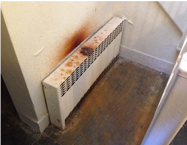
Rusty radiator unit cover
