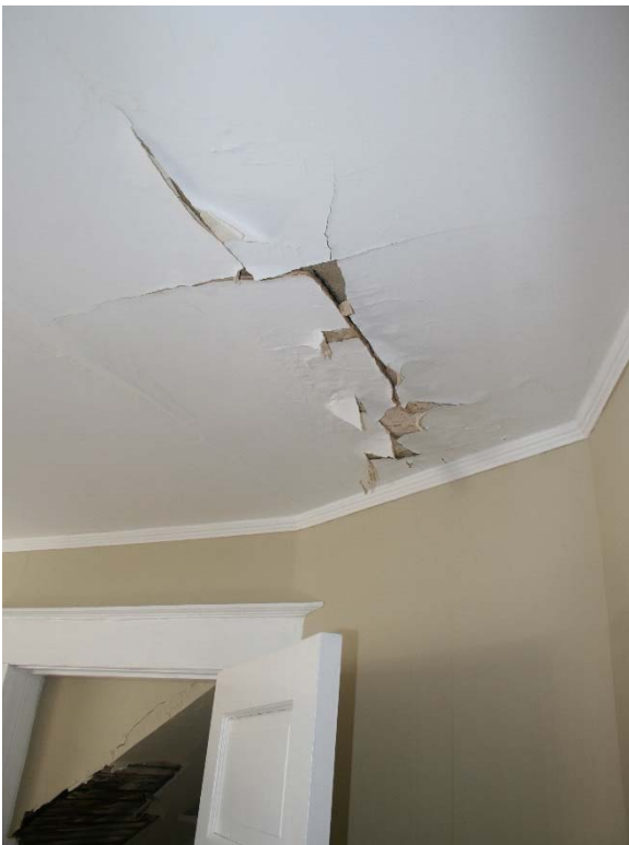
Evidence of water damage in upstairs bedroom ceiling
