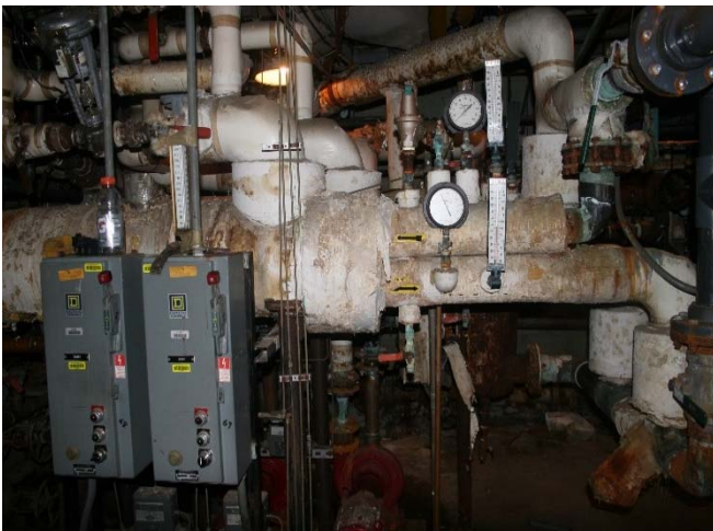
Hot water supply piping and electrical components
