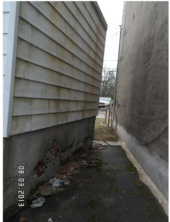
Close up image of foundation failure and narrow alleyway between adjacent structure
