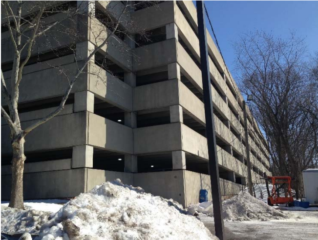
View of rear of parking structure. Area used as storage for trailers.
