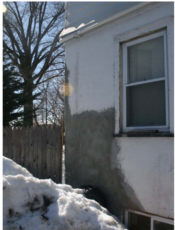
Rotting windows sill and evidence of recent stucco repair
