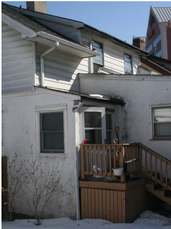
View of rear entrance to property, evidence of water damage along wall face, missing gutters and roof liters
